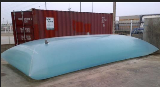
Testing facility with water storage tank
